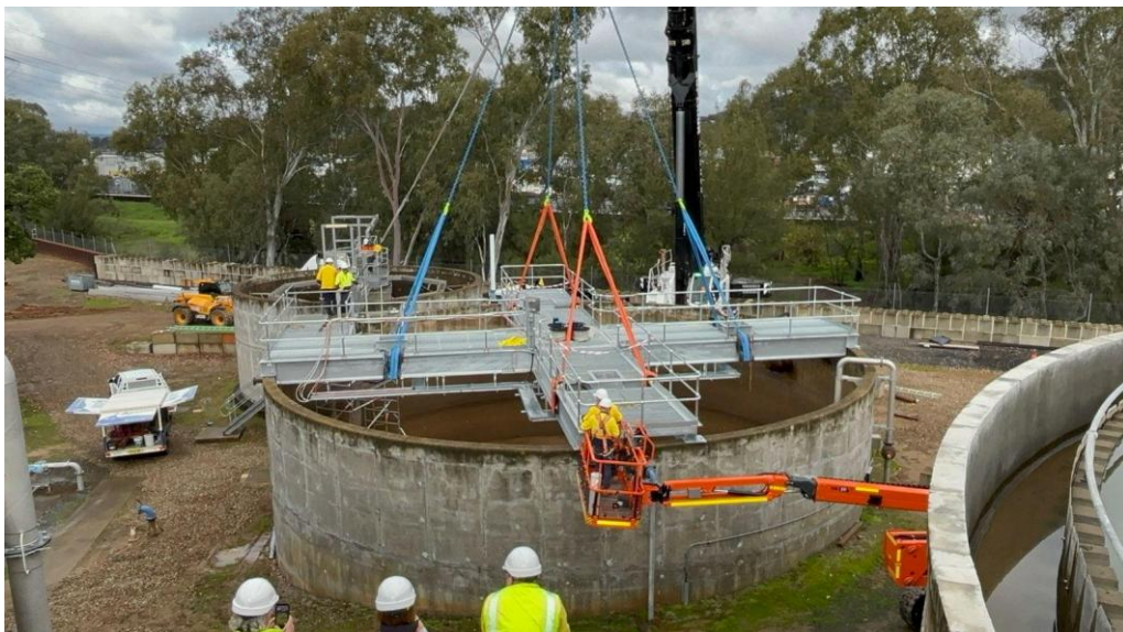
Figure 5: Bridge installation as a single lift
