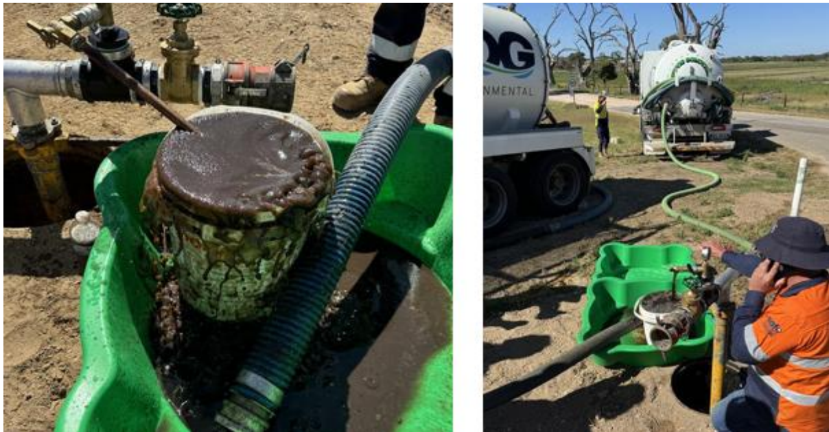
FIGURE 5: DISCHARGE AND COLLECTION OF THE DIRTY ICE
