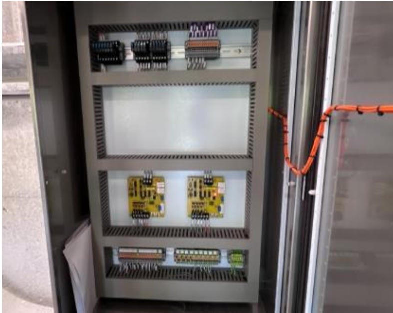
Figure 4 Lime AirSweep® marshall panel built by Ventia SCAS Services
