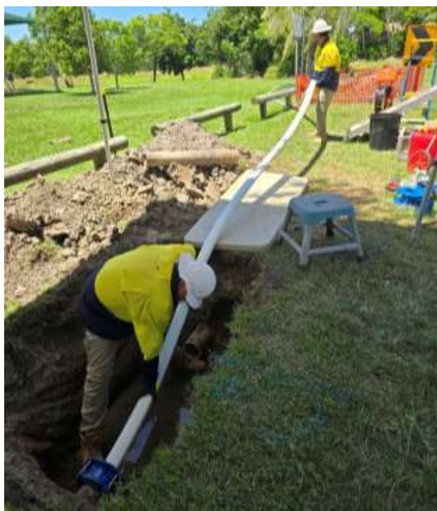
Figure 7: The construction footprint for the installation of the Primus Liner DN150 is extremely small.
