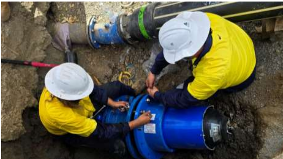
Figure 5: Installation of the Primus Line end connector at the Hope Island Road entry pit. The blue connector body provides the mechanical and pressure-tight transition between the Primus Liner and the existing flanged network connection.
