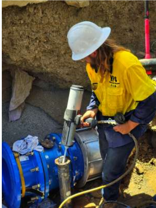
Figure 6: A Primus Line DN400 PN16 R connector was chosen for the installation. Though flanges it connects on side back to the host pipe and on the opposite side back to the existing pipeline system.
