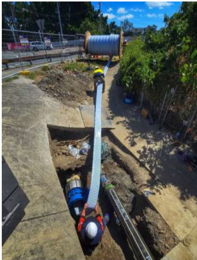
Figure 2: Primus Liner being pulled from the transport reel into the access pit during the Hope Island Road installation. The compact reel and minimal site footprint are characteristic of the system.
