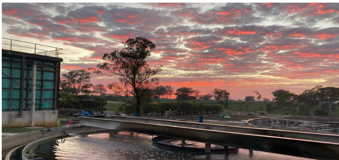
Figure 3 — Gatton STP at dawn, showing primary clarifiers. Operators monitored lagoon levels and assessed release conditions before sunrise throughout the incident period daily.
