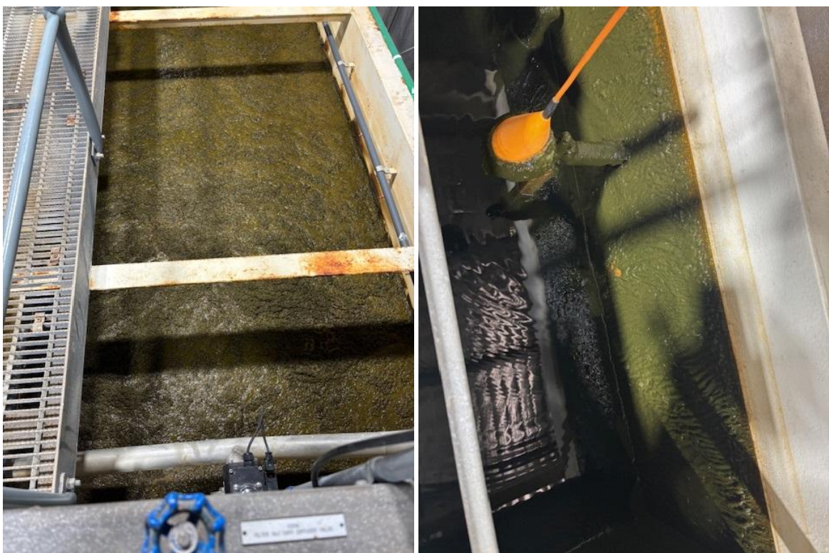
Figure 4. Rainbow WTP dissolved air flotation filtration (DAFF) process affected by green algae.
