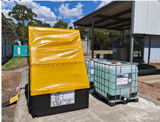
Figure 6 - Setup of site trial to dose Calgon T in Rosslynne WTP post-filtration and pre-chlorination
