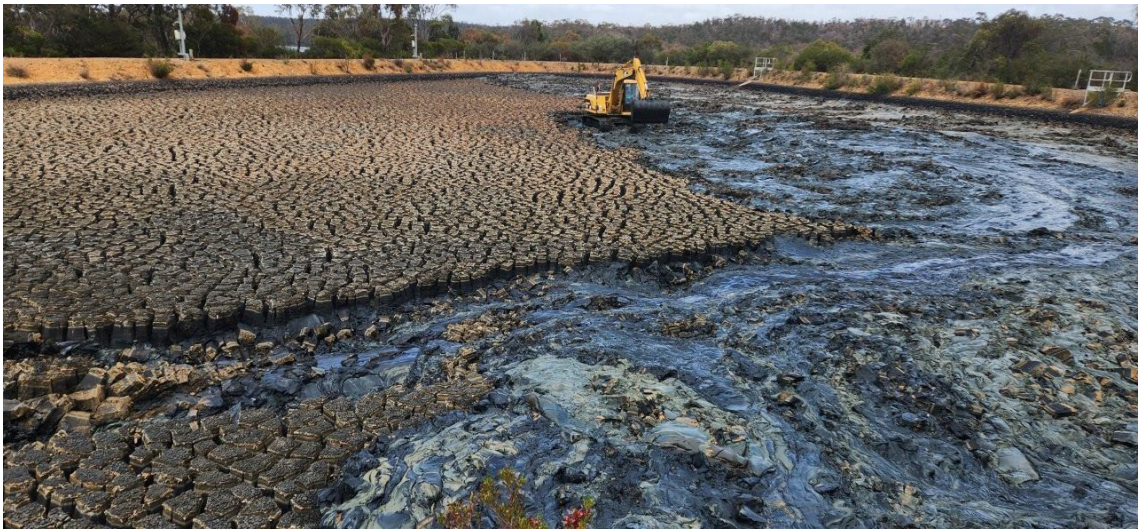
Figure 10: Lagoon 2 being turned over
