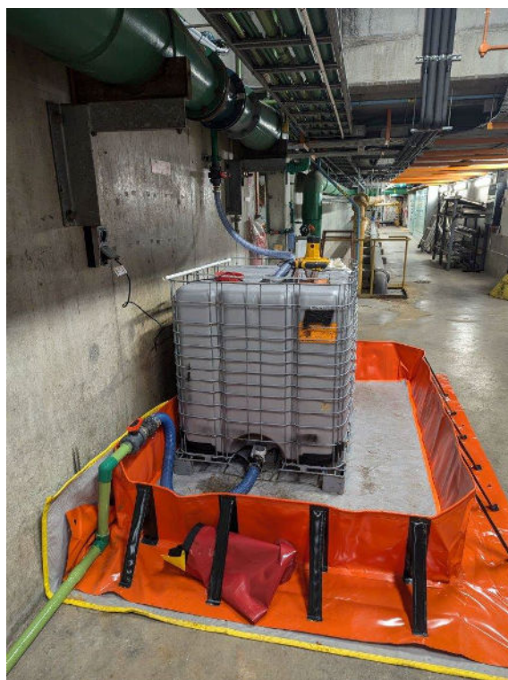
Figure 8: Temporary poly batching system
