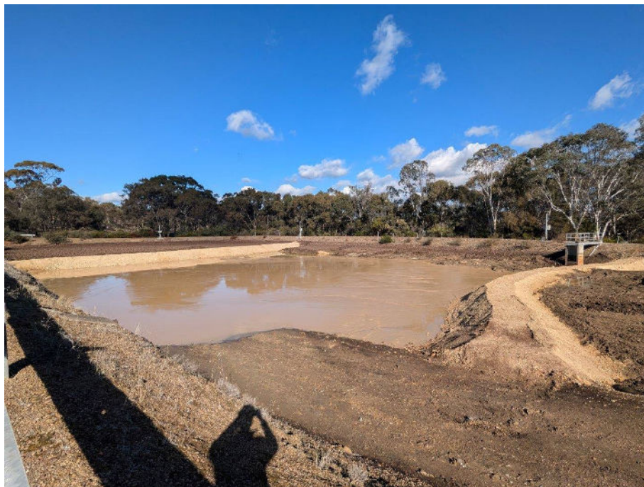
Figure 7: Earthen embankments installed to Lagoon 1
