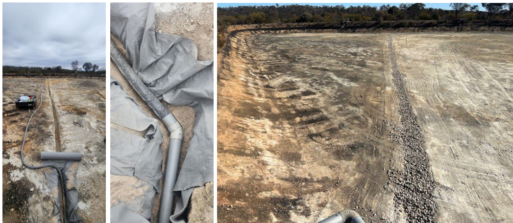
Figure 11: Underdrain pipe installed to base of Lagoon 2
