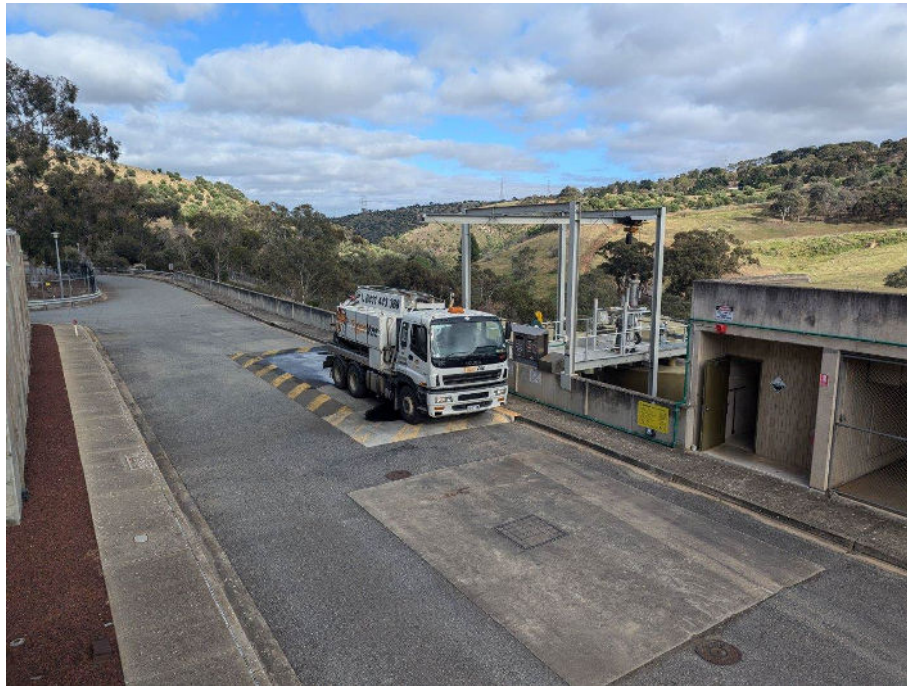
Figure 12: Vacuum truck unloading sludge at Little Para WTP
