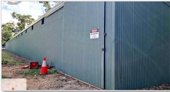
Figure 1. External shed structure
