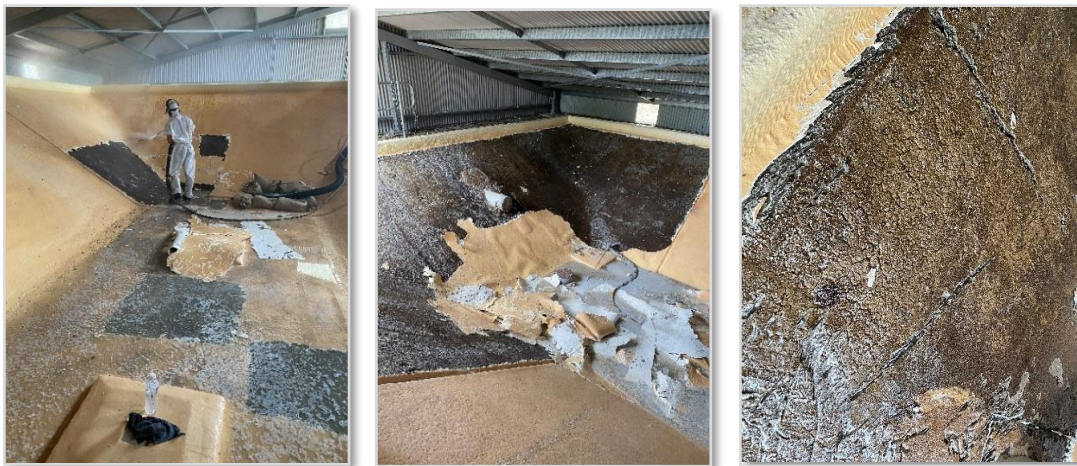
Fig. 4-6: Removal of polyurea coating from basin
