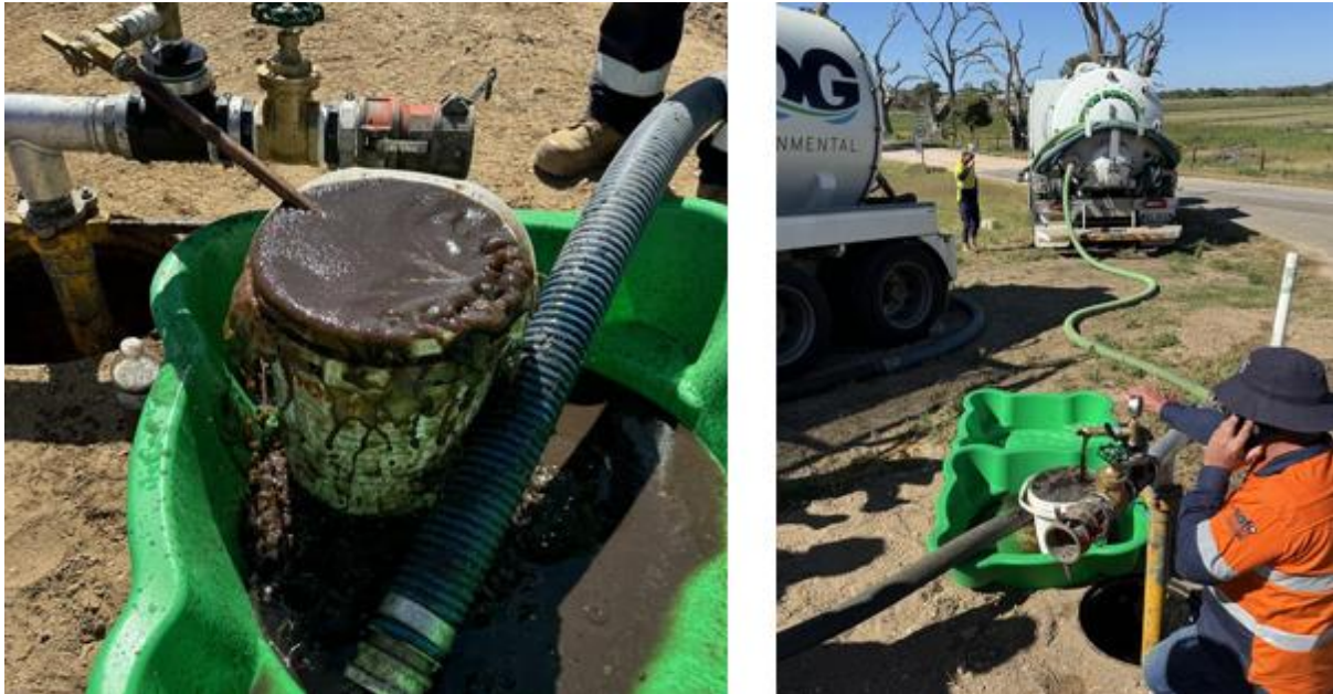
FIGURE 5: DISCHARGE AND COLLECTION OF THE DIRTY ICE
