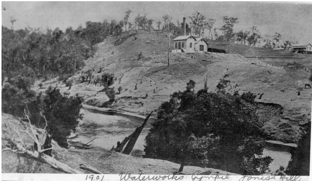
Figure 1 - Jones Hill Waterworks, 1901
