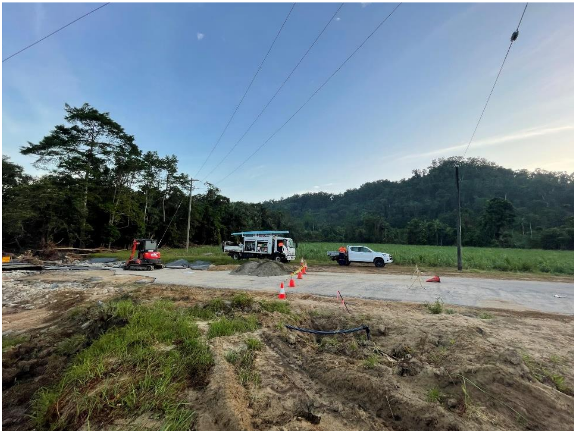
Figure 3 – Repairs underway, Mossman Qld.
