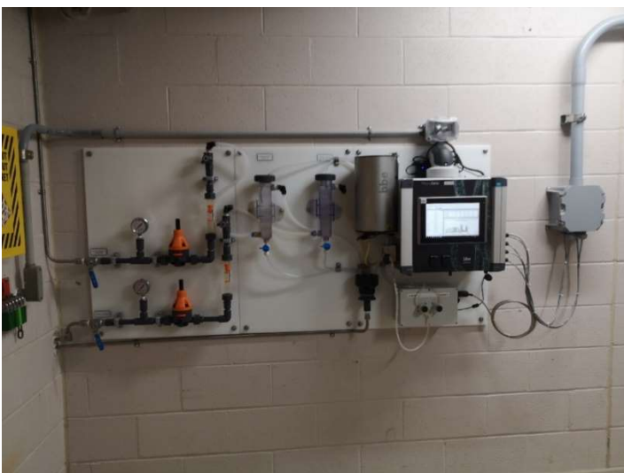
Fig. 8: Example of an AlgaeOnlineAnalyser at the water treatment plant in Toronto
