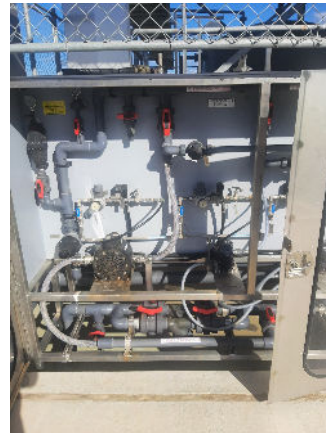
Citric Acid Dosing Cabinet with multiple equipment at ground level
