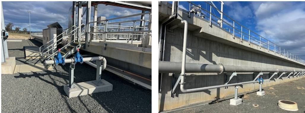
Suction pipework on Anoxic Zones 1 and 2 at Cessnock WWTW
