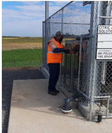
Citric Acid Dosing Cabinet with multiple equipment at ground level
