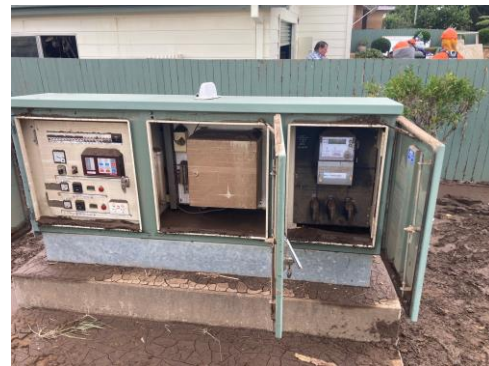
Figure 6 - Inundated SPS Switchboard
