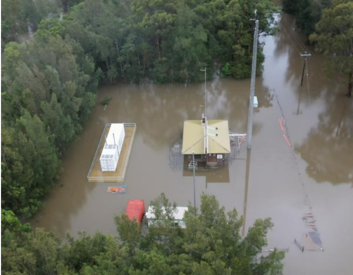
Figure 7 - Taree SPS #6 - Flooded over the floor height but still operational & refueling the generator
