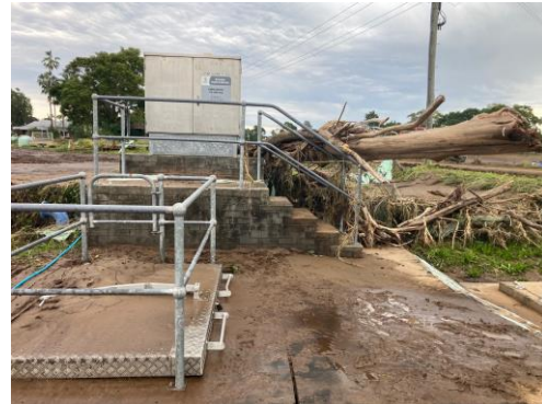
Figure 5 - Taree SPS#4 - Flood Rack & Mud
