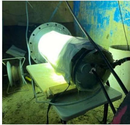
Picture 2: Curing of the SAERTEX-LINER®
