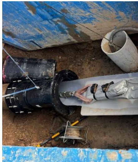
Picture 1: CIP JOINT of NovaSiria® mounted on the host pipe
