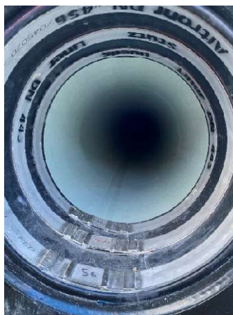
Picture 3: Installed Liner and Liner End Seals
