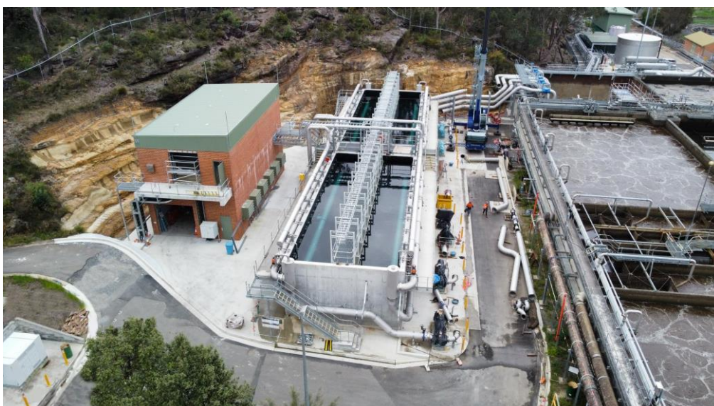
Figure 8: Winmalee STP, New South Wales. SBR plant converted to MBR in 2024.
