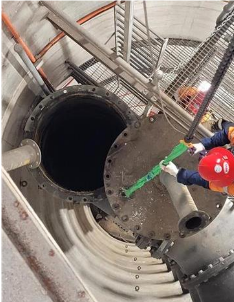
Figure 5 Blanking plate at intake tower
