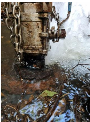
Figure 1 Leak at injection point
