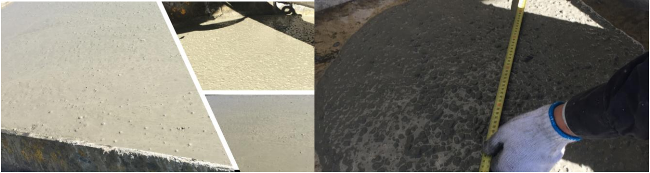
Figure 3: Concrete with CNT additive, measuring the spread using the slump test.
