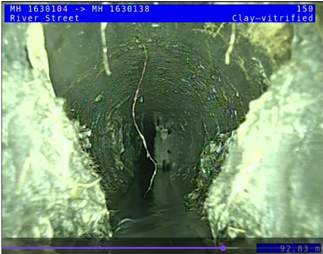
Figure 4: Example of CCTV Footage showing asset prior to cleaning
