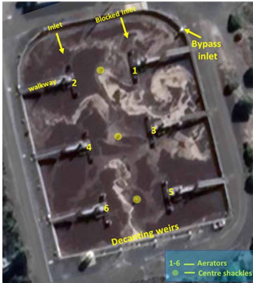
Figure 1: The IDEA Basin at Finger Point WWTP
