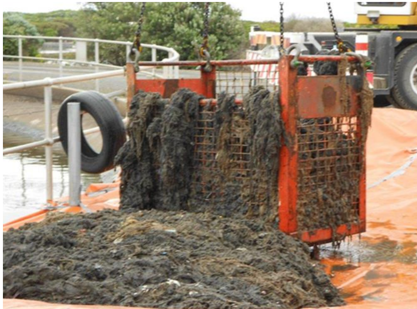
Figure 2: Material lifted out of the basin in 2013
