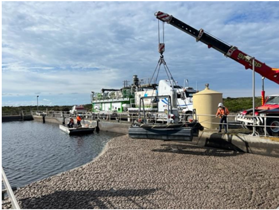
Figure 5: The robotic dredge being launched into the basin
