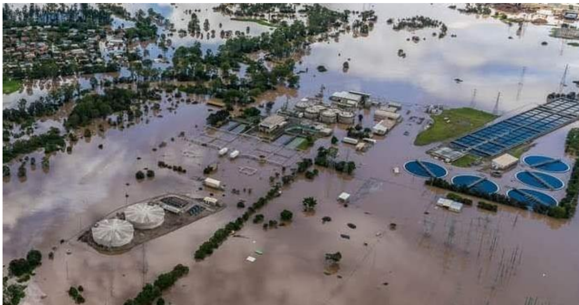
Figure 1: Aerial view of the flooded treatment plant and surrounding area
