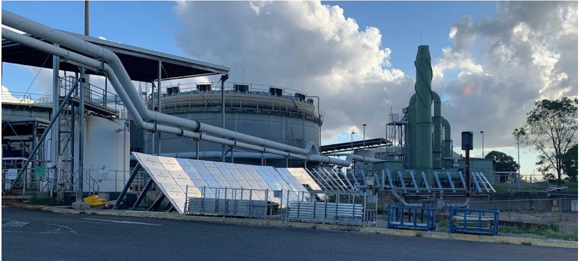
Figure 3: Flood barrier during assembly at Oxley RRC
