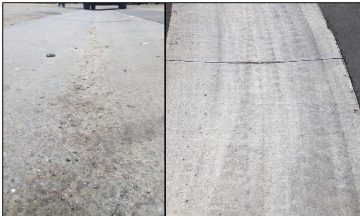
Figure 7: Concrete Company C Project – Town home Drainage (December 2017; 31-months old); Reference (Left) and CNT Additive (Right)
