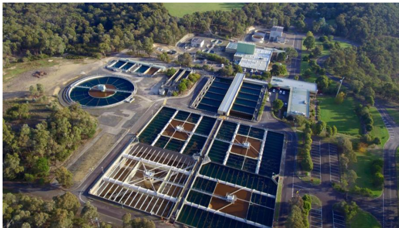
Figure 1: Winneke Treatment Plant, Clarifiers & Filters
