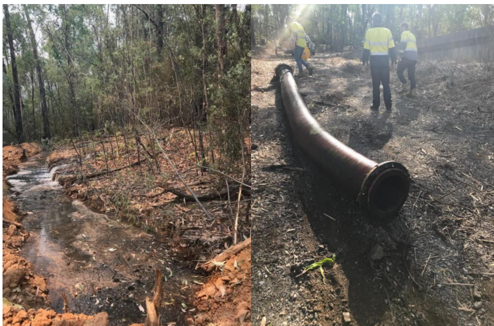
Figure 3: The silt terrace and the discovered flexible offtake.
