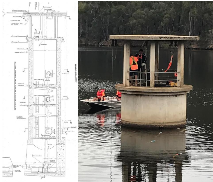
Figure 1: The construction drawings of the Loombah offtake tower – circa 1940, and the standing platform of the tower.
