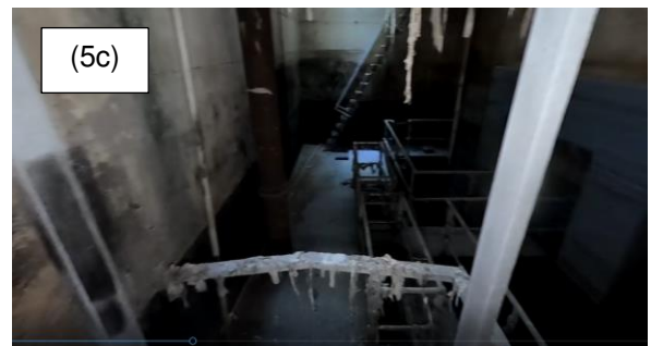
Figures 5a to 5c: The Go-Pro camera was lowered from the main surface landing into the wet well via the bar-screen opening (5a). The camera was able to provide incredible 360-degree footage of the DN1500 gravity sewer (5b) and the wet well intermediate landing (5c).
