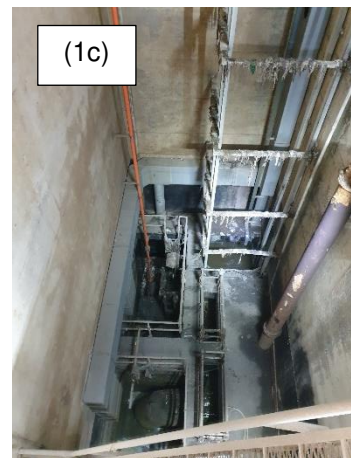
Figures 1a to 1c: The Loganholme lift station is comprised of a 20m deep dry/wet-well arrangement with a pumping capacity of in excess of 3,500L/s
