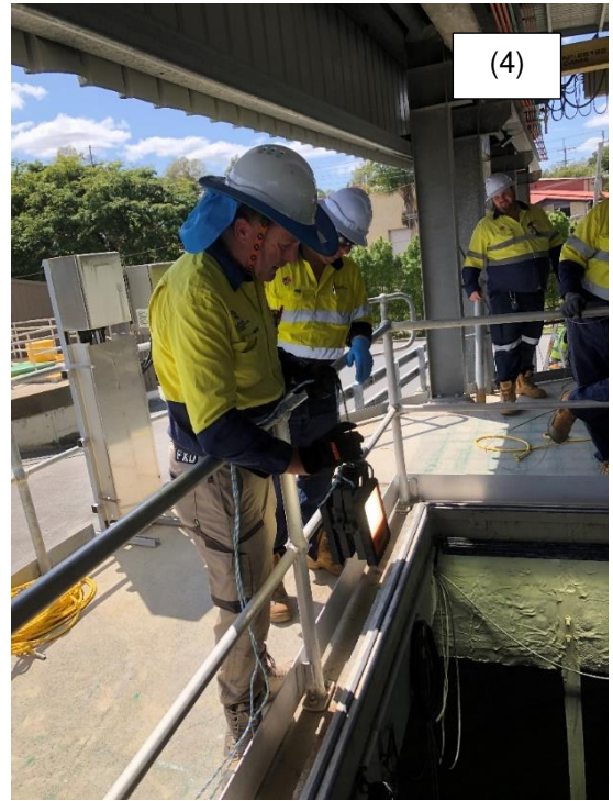
Figure 4: Example of the Go-Pro 360 camera being lowered into a confined space
