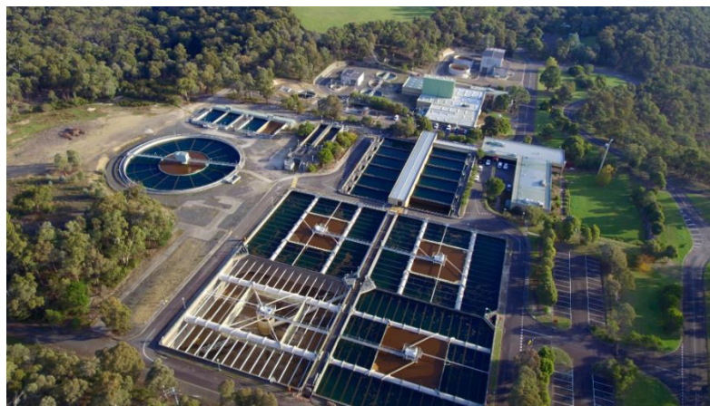
Figure 1: Winneke Treatment Plant, Clarifiers & Filters
