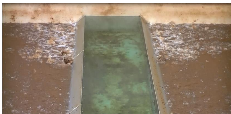
Figure 3: Boiling occurring due to rapid onset of the washwater pumps
