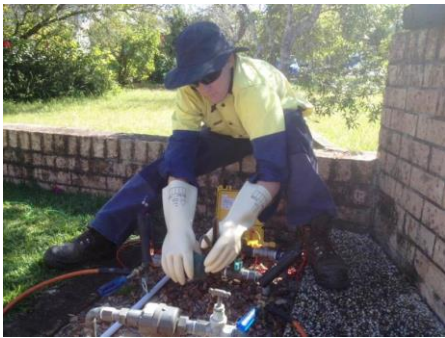
Photo 5: Construction: replacement of aging infrastructure and construction for future growth
