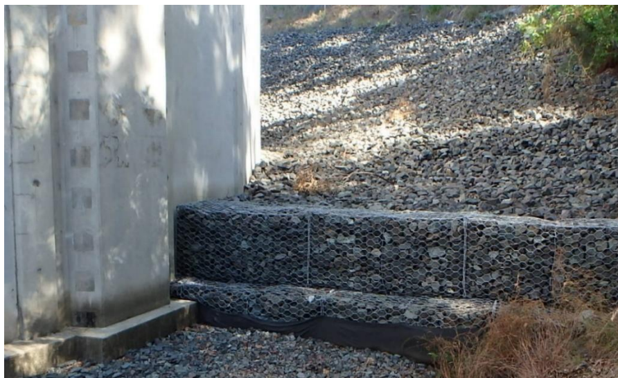
Figure 6: Using the tank walls to retain the embankment area
