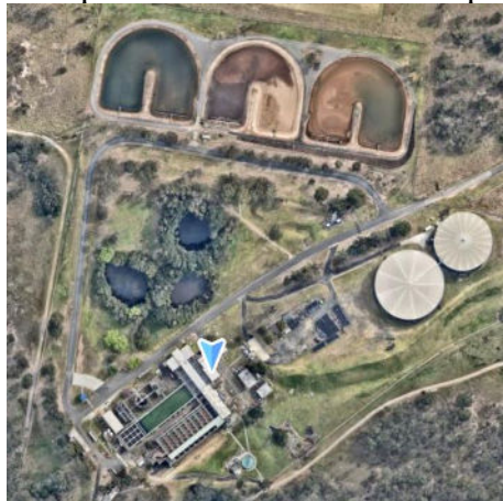
Figure 1: Orchard Hills Water Filtration Plant and residual drying lagoons
