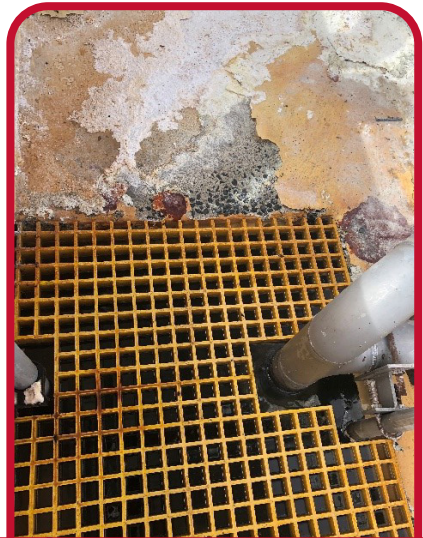
Powdered soda ash created a hazard as it would create an exothermic reaction inside the bund.
