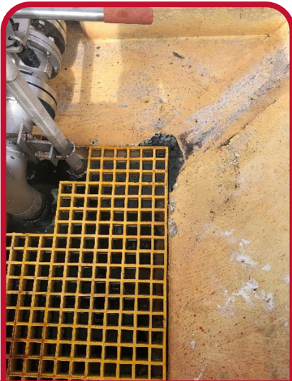
Powdered soda ash created a hazard as it would create an exothermic reaction inside the bund.
