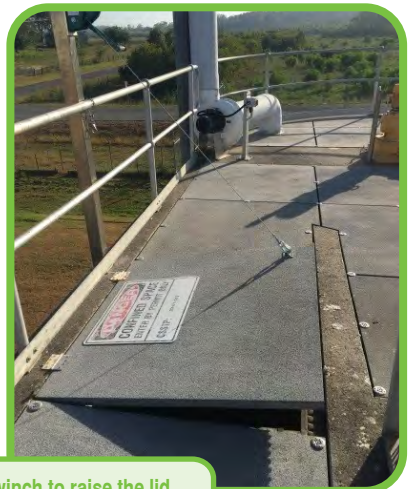
Winding the hand winch to raise the lid.
