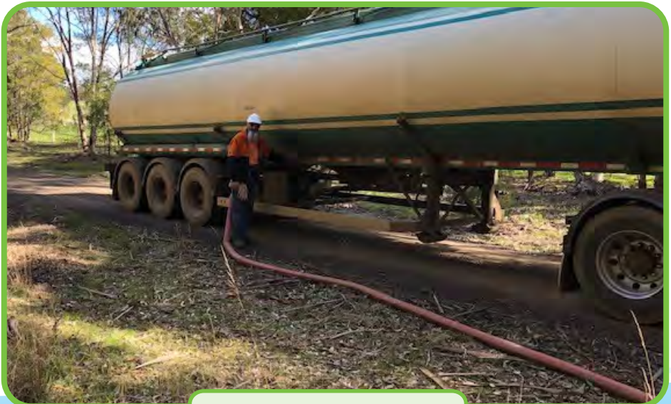
Tanker connected to the main.
