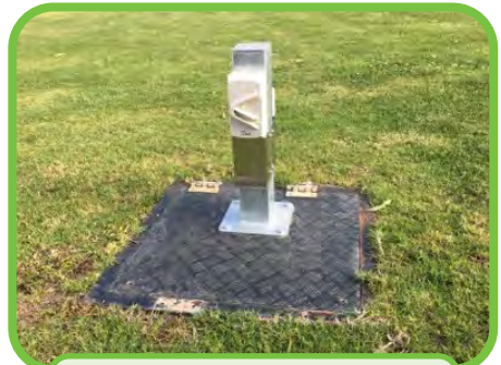
Relocated Switches outside of the tank.
