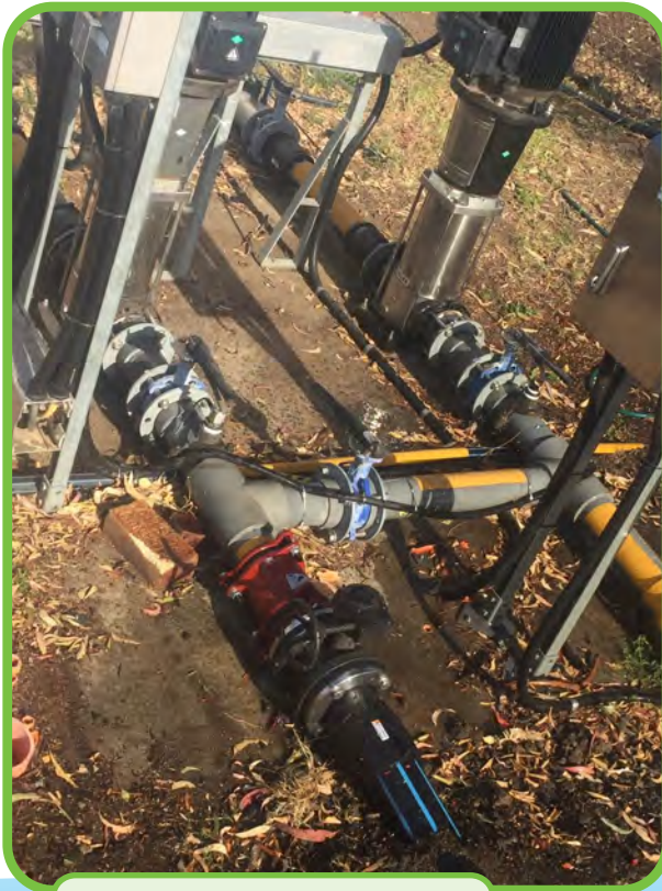
After the new pipework was installed.
