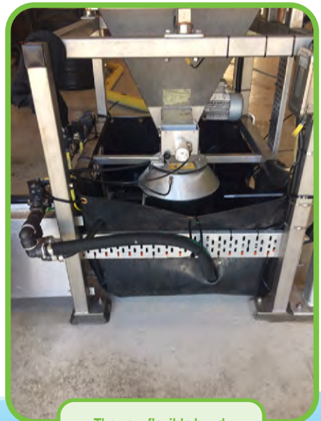
The new flexible bund.
