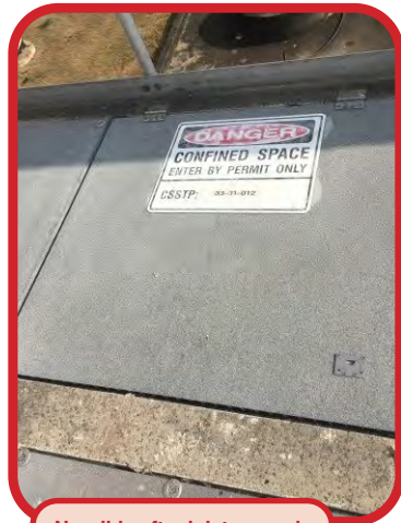
New lids after inlet upgrade.
