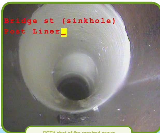
CCTV shot of the repaired sewer.
