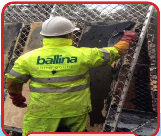
Manually cleaning the membranes.
