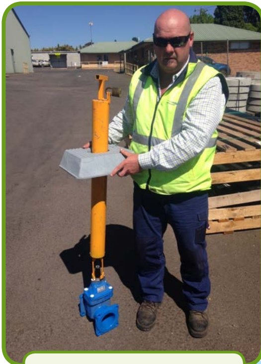
The valve locking clamp.
