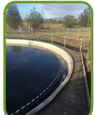
The rubber footings at the base of the handrails to stop animals getting in.
