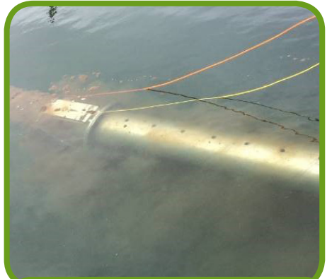
A partly cleaned launder.
