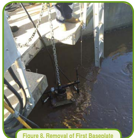
Figure 8. Removal of First Baseplate Attached to Jib Crane
