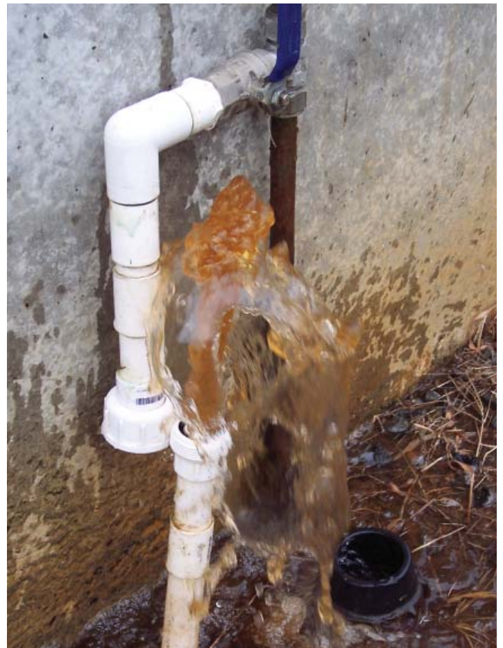
▼ Flushing dirty water sample lines.
