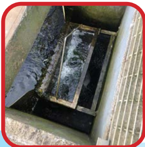
Clarifier outlet filter baskets and UV system blocked up by solids build
