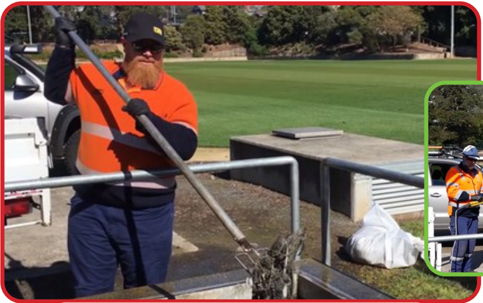
Manual removal of rag from sewage pump stations.
