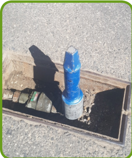
The stoptap removal key fitted onto the stoptap.
