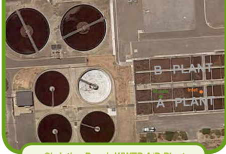
Christies Beach WWTW A/B Plant and Ammonia analyser location
