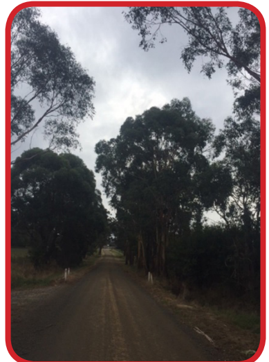
Remote water main with one customer at end of 7-8km 100mm main
