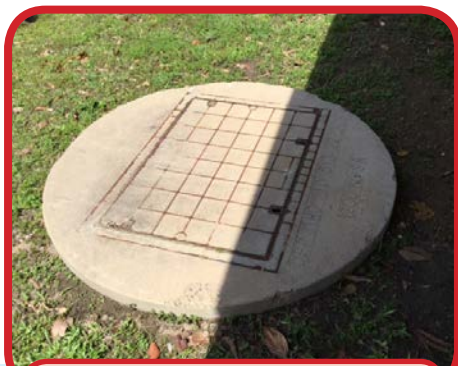
Example of a concrete gatic lid, typically used by Power and Water Corporation
