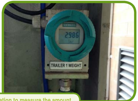
Pressure measurement installation to measure the amount of sludge loaded into trailers.
