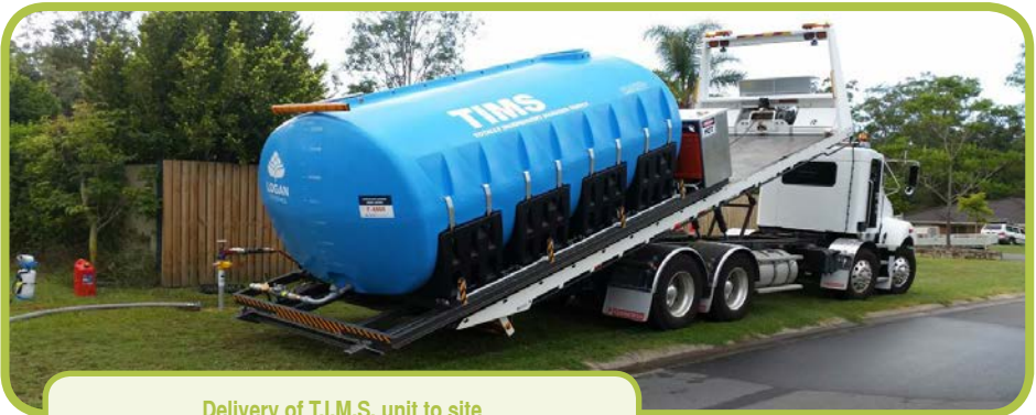
Stanmore Road T.I.M.S. deployment during flood repairs
