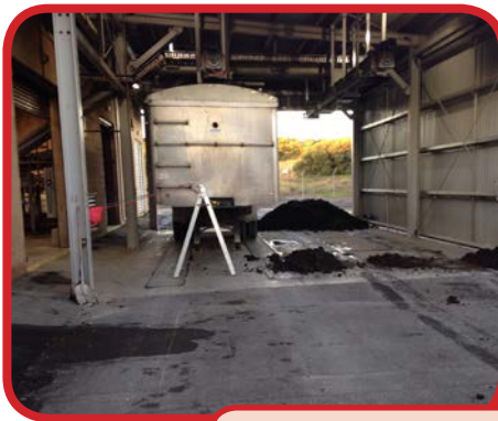
Examples of the OHS and spillage problems at the IDEA sewage treatment plant at Warrnambool
