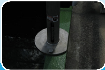
Pedestal internal drive shaft
