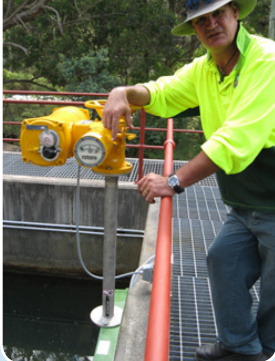
The penstock extension
