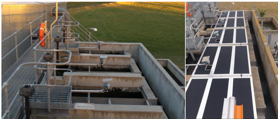
Figure 2: Kyneton BACs - (L) before covers, (R) slip-in fly screen covers
