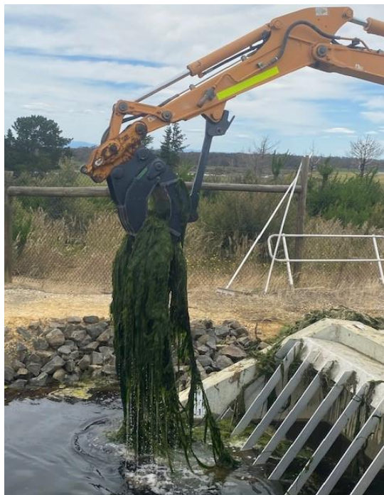
Figure 2: Mechanical removal of weed & algae at ROS Channel - Peg 54 Bar Screen
