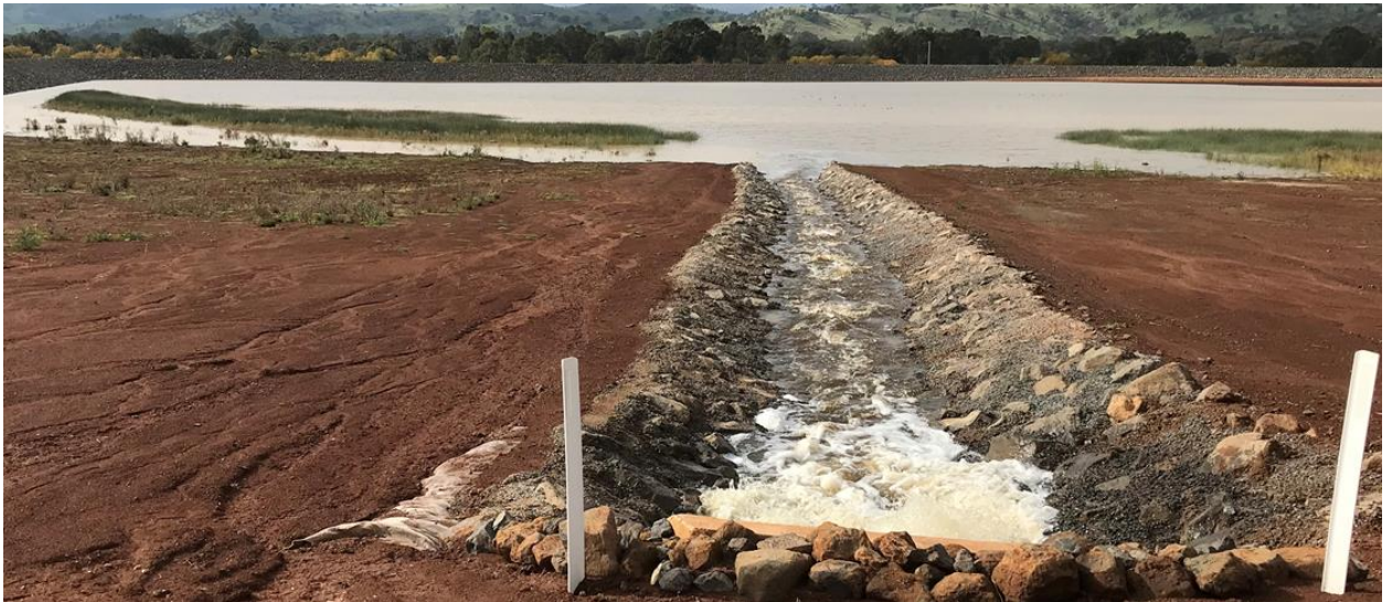
Figure 2: Planned Work - Dam Safety Inspections
