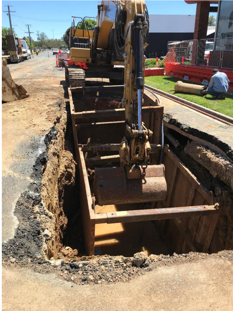
Figure 3: Reactive Work - Sewer leak repair
