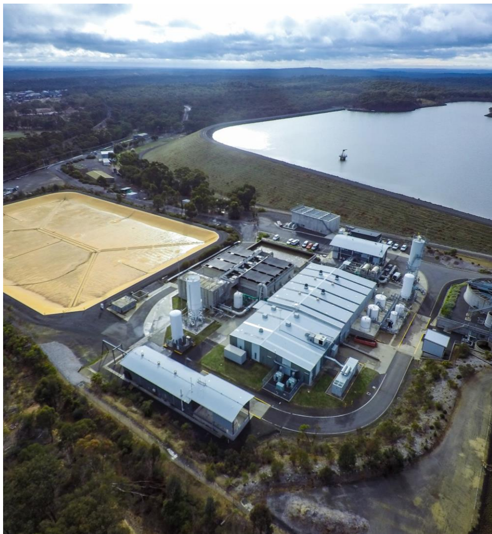
Figure 1: Sandhurst Reservoir and Water Treatment Plant
