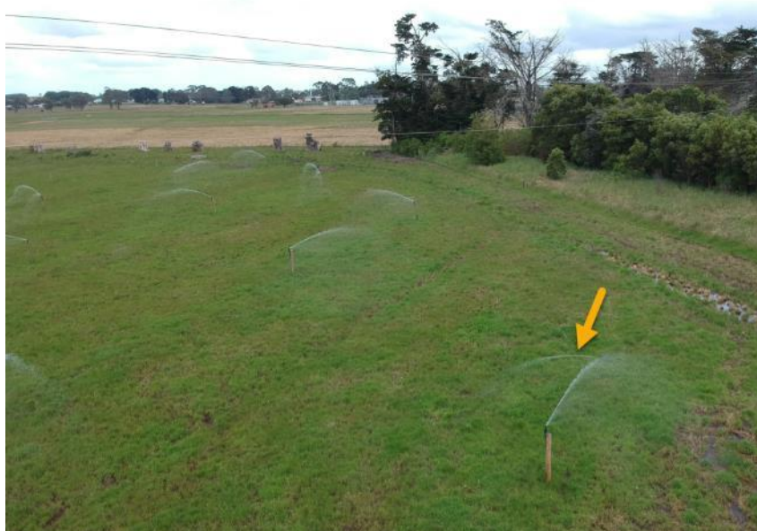
Figure 4: Drone monitoring and sprinkler missing a post (arrow)
