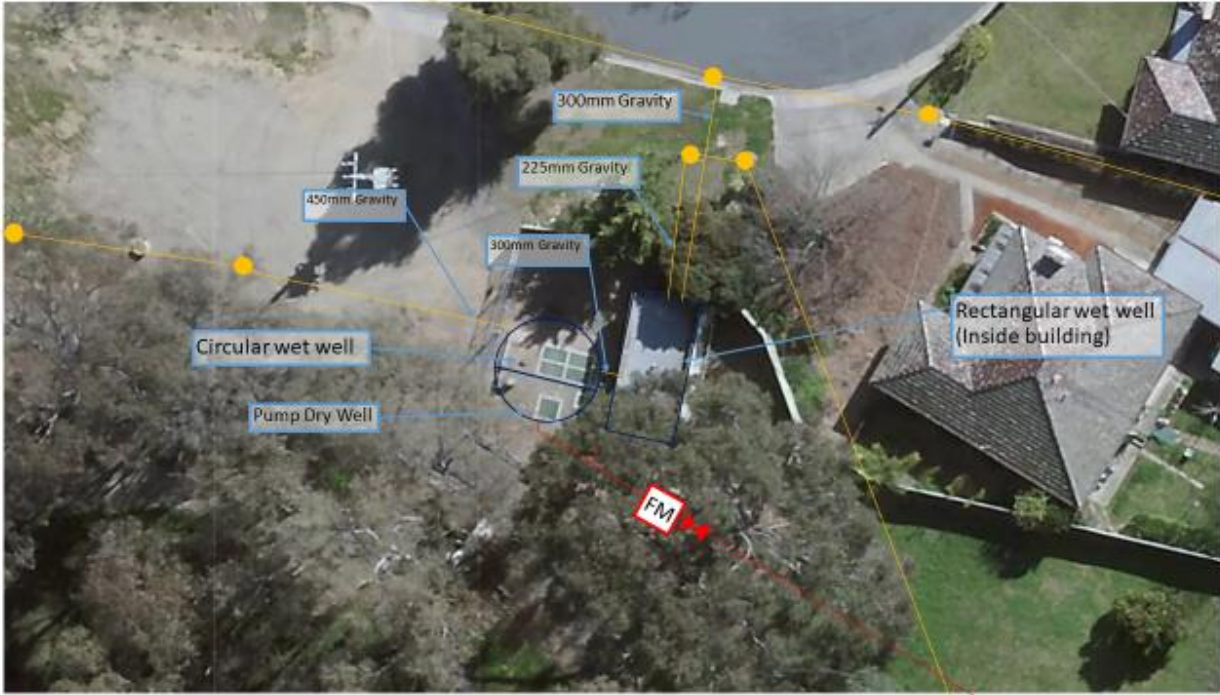
Figure 1: Aerial view of the Swan Street Sewer Pumps Station
