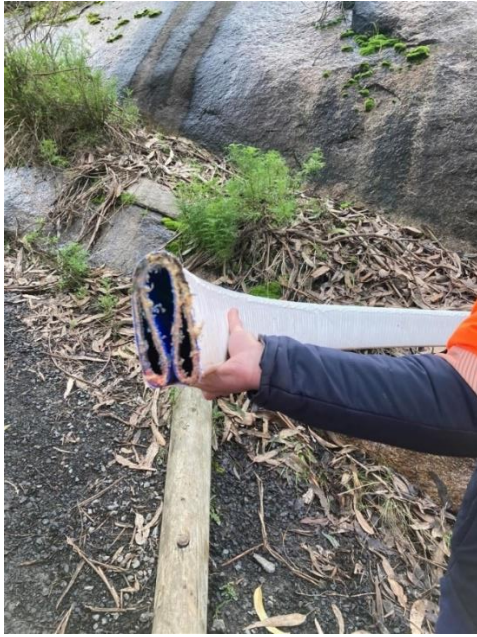
Figure 4: Primus Line in a compressed 'C' shape for installation
