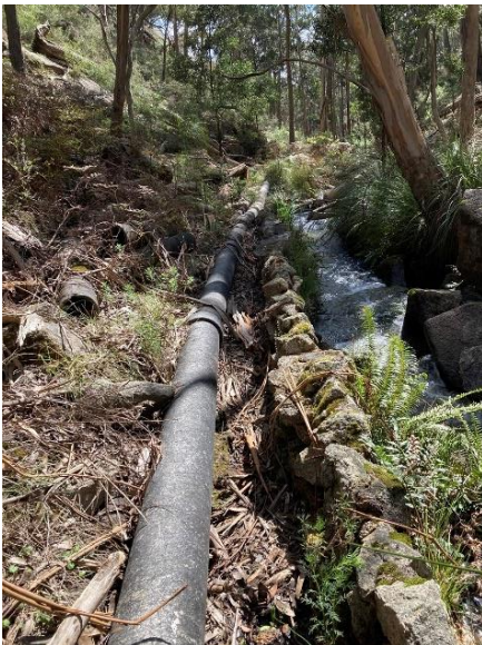
Figure 1: Mt Cole Pipeline - DN250 AC (Asbestos Cement) Section
