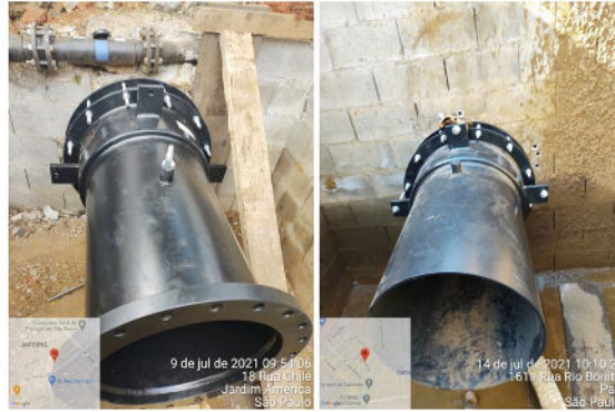
Picture 5. CIP JOINTS
