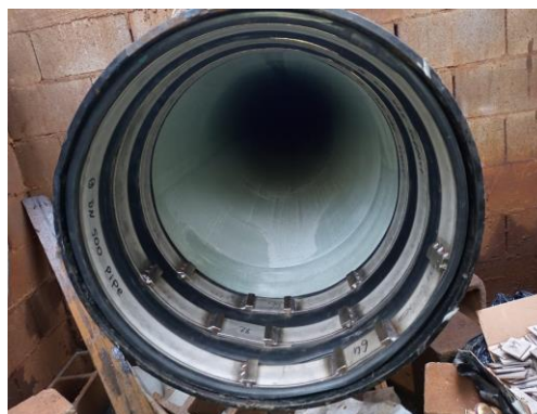
Picture 3. Installed Liner End Seal
