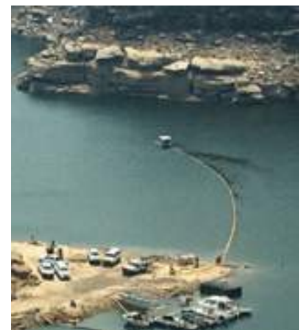
Figure 4. Installation of a boom in a fire affected reservoir.
