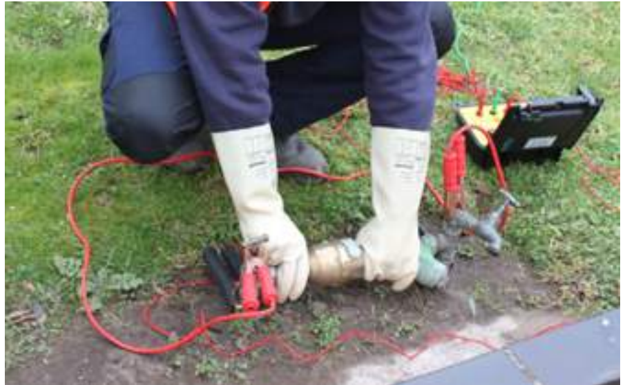
Figure 3. Correct safety practices in use to reduce electrocution risks. The red clamps are the bonding strap and the black clamps are for the Plumb Guard. The other black clamp is attached to the water pipe near the operator's left hand.
