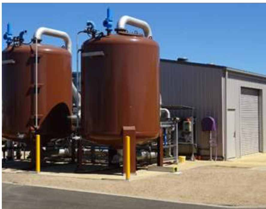
Figure 5. Pressure filters at the WWTP.
