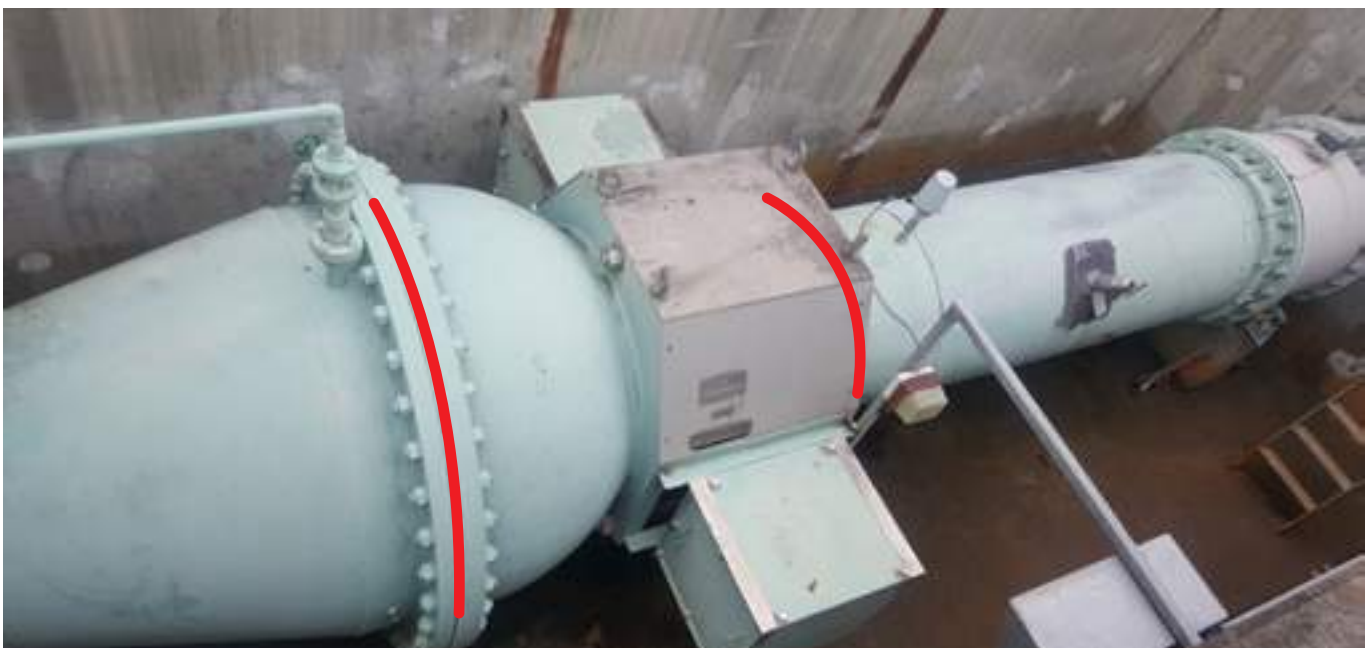
Figure 1. The Raw Water Inlet Flow Control Valve (GKILR 800). The two curved red lines indicate the flange faces of the existing GKILR and the space the new/engineered solution had to fit into.
