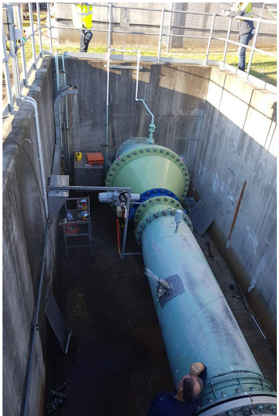
Figure 3. The temporary valve 'in position' and operating successfully.
