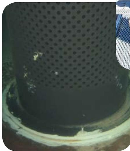
the uneven concrete surface. The screen was fitted by divers using an air-powered drill to place 16mm SS tru-bolts through the base flange and into the concrete floor. The tru-bolts were dipped in NMP 1720 epoxy to seal them into the concrete and avoid future 'Crevice corrosion'. The base flange area was also sealed to the floor using 1720 epoxy with good results.
