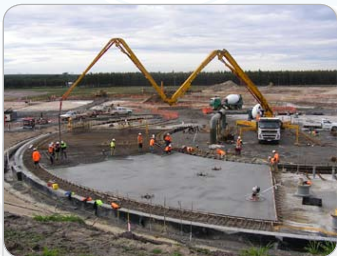
"The first quarter of the membrane bio reactor base at the Gippsland Water Factory being poured in late July"
