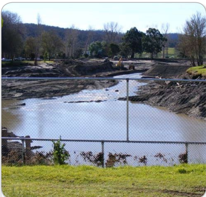
“The dewatered pool at Cowwarr undergoing rehabilitation works”
