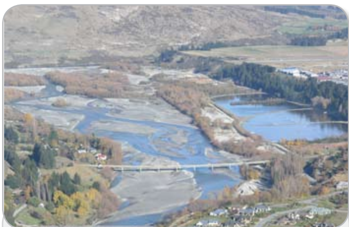
The Shotover River in Queenstown and the WWTP on the right.
