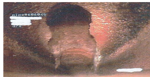
The photo above is a "cavity" in a 600 diameter sewer main.
